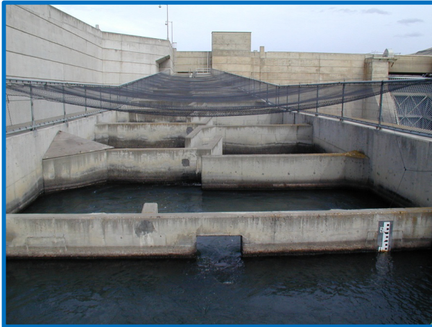
Figure 1. Design of the John Day Dam north ladder flow control section as seen from the count station catwalk in 2009. Overhead netting placed to keep fish from jumping out of the ladder.
